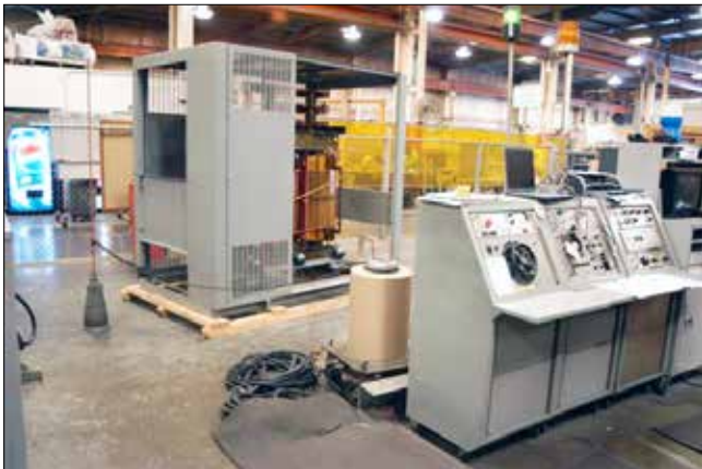
Figure 21. Final test area for Medium-Voltage transformers.
