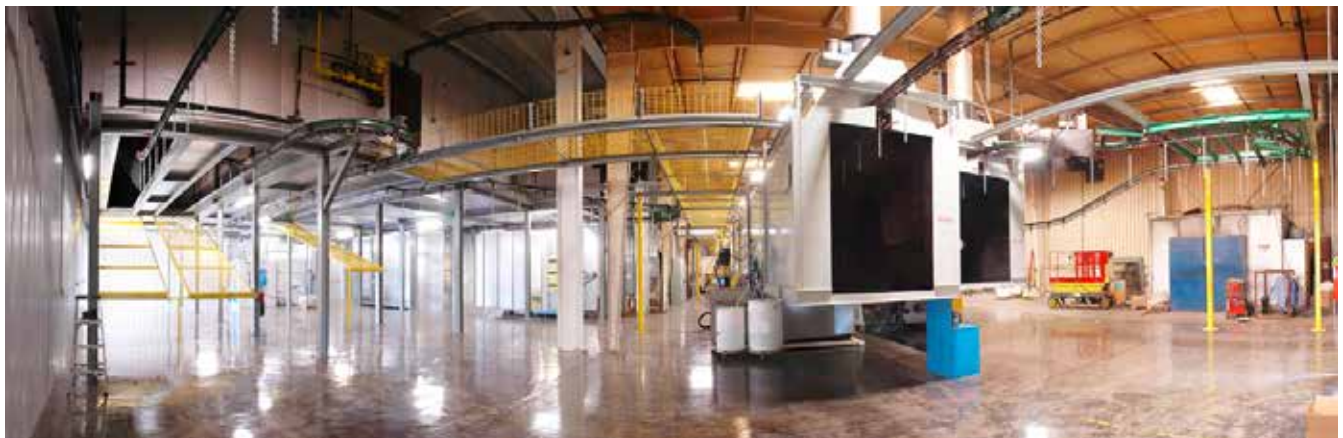
Figure 18. Powder coat paint facility.
