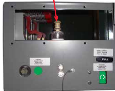
Figure 6. Views showing closed position of In-Line visible disconnect at left and open position of In-Line visible disconnect at right. Also shown are position-indicator targets for visible disconnect and vacuum interrupter along with the pull handle used to reset the magnetic latch that initiates tripping of MAVriC ® when an overcurrent occurs. CTs on outgoing cables sense the overcurrent; the Self-Powered Relay processes the overcurrent condition and sends signal to release the magnetic latch; the plunger of the magnetic latch engages the trip lever on the MAVriC ® to separate the monostable magnetic actuators, breaking the magnetic field and releasing the spring energy to open/close the vacuum-interrupter contacts.
