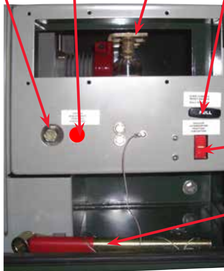
Figure 6. Views showing closed position of In-Line visible disconnect at left and open position of In-Line visible disconnect at right. Also shown are position-indicator targets for visible disconnect and vacuum interrupter along with the pull handle used to reset the magnetic latch that initiates tripping of MAVriC ® when an overcurrent occurs. CTs on outgoing cables sense the overcurrent; the Self-Powered Relay processes the overcurrent condition and sends signal to release the magnetic latch; the plunger of the magnetic latch engages the trip lever on the MAVriC ® to separate the monostable magnetic actuators, breaking the magnetic field and releasing the spring energy to open/close the vacuum-interrupter contacts.
