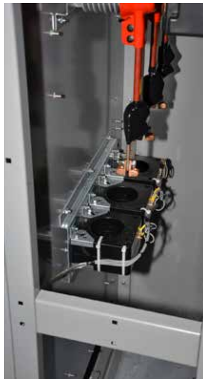
Figure 6. Three (3) 4.16kV voltage transformers are furnished in each incoming termination compartment (Bay 1 and Bay 19). Each set of VTs provides voltage sensing input to the power monitoring unit in the associated main incoming fused switches, which are in Bay 2 and Bay 18. The voltage input combined with the current input allows the meter to produce all of the associated measurements: phase voltage, line-to-line voltage, average voltage, power factor, kW, kWh, etc.
