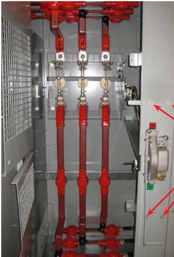
Figure 11. The Auto-jet® II Load-Interrupter Switch (rated 600-amperes continuous) in Bay 11 is the bus-tie switch between the two incoming sources that enter the switchgear through Bay 1 and Bay 19. If either source is lost, the associated main fused-switch is opened, non-critical loads are shed, and then the bus-tie switch can be closed to pick up the most critical loads on each bus section. Key interlocks among the switches in these three (3) bays insure that the sequencing of opening and closing the various switches is matched to the ability of the remaining circuit to carry the connected load.
