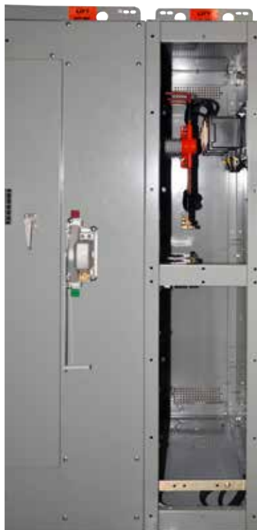
Figure 6. Three (3) 4.16kV voltage transformers are furnished in each incoming termination compartment (Bay 1 and Bay 19). Each set of VTs provides voltage sensing input to the power monitoring unit in the associated main incoming fused switches, which are in Bay 2 and Bay 18. The voltage input combined with the current input allows the meter to produce all of the associated measurements: phase voltage, line-to-line voltage, average voltage, power factor, kW, kWh, etc.
