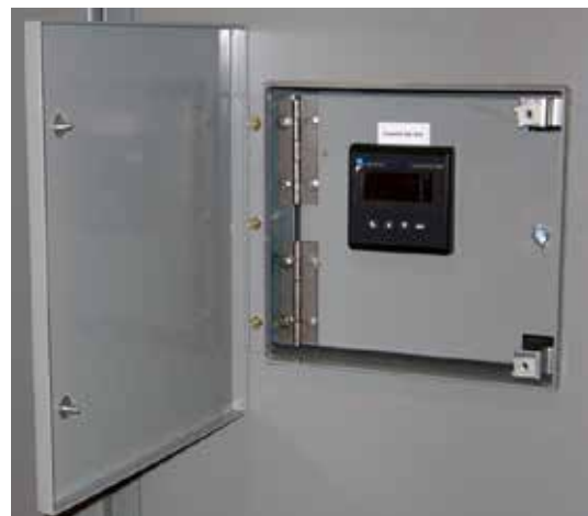
Figure 5. Pictured above is Bay 4, which includes the feeder switch and current-limiting fuses for switching and protection of the load feeder circuit. Inset (at top right) shows steel perforated screen that is encountered over the switch when the enclosure door is opened and that allows access to the fuses without exposure to the switch terminals; and (at bottom right) the digital power monitoring meter that allows real-time display of the various circuit parameters. The power monitor is mounted on a hinged, bolted panel in a low-voltage compartment that is isolated from high voltage. The operating handle on this bay is painted red to differentiate it from the handles of the incoming switches.
