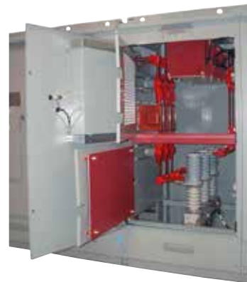
Figure 15. Pictured above is Bay 3, which includes the VBT vacuum interrupter switch for frequent sustained switching of the load circuit.
