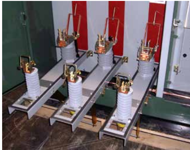
Figure 10. Federal Pacific has developed a new turnbuckle, which is connected between the fuse panel and the red GPO-3 fiberglass shutter barrier. The enhanced design (in black) has increased mechanical capability and is easier to install, remove and replace. It can be used to replace installed earlier-design turnbuckles, requiring only the addition of a suitably-sized hole in the barrier.
