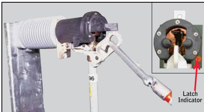
Figure 1. Closed: Positive Latch Indicator Extended (see inset). Hookstick Ready To Open.
