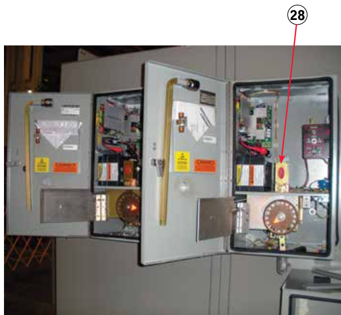
Figure 8. Open door view of Fast-Trip Style Type PM Motor Operator showing motor and decoupler lever.
