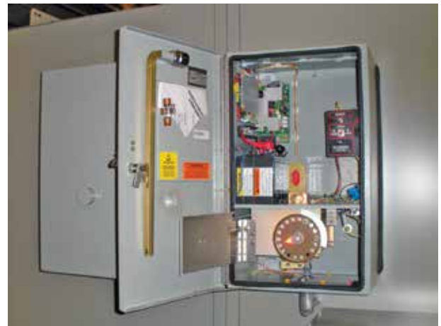
Figure 8. The Fast-Trip Motor Operator is illustrated above with the interlocked cover over the motor shown closed in the photo at left and with the cover open in the photo at right. As the motor rotates at high speed, if the cover is open motor operation is suspended. A separate key interlock (see arrow in photo) can be provided to block operation of the motor operator for other specific requirements, such as requiring that all switches be open before allowing access to fuses.
