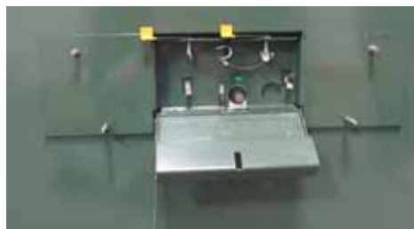
Figure 2. PROM-PM Mounting Plate on PSI/II
