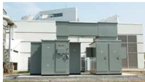
Figure 3. Automatic-transfer switchgear with Fast-Trip Transfer motor operators is pictured in the photo above. Transfer to the alternate source is achieved in approximately twenty (20) cycles.
