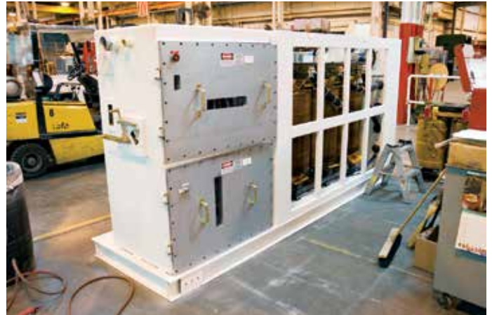
Figure 10. An enclosed dry-type transformer with controls housed in an explosion proof permissible housing are applied for operation of heavy mining equipment.
