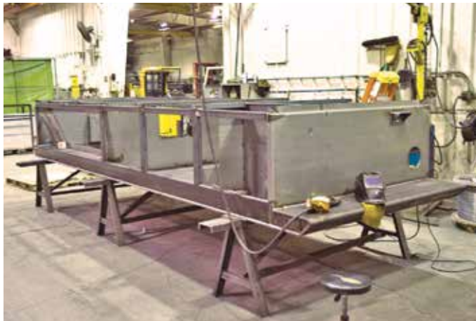
Figure 1. Welding operations utilize certified personnel and superior materials.
