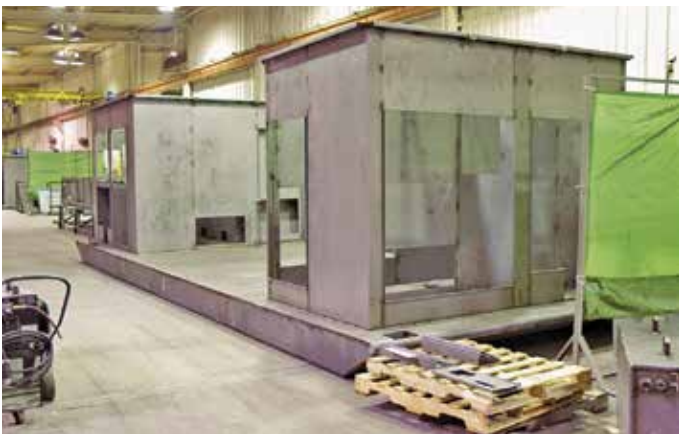
Figure 3. Large superstructures are cleaned to remove all oils and dirt prior to painting.
