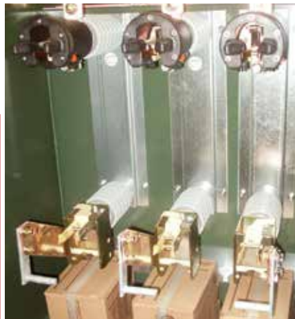
Figure 5. Lubrication points on loadbreak fuse mounting include three contact locations, namely, the main contact, forward contact and fuse hinge contacts.
