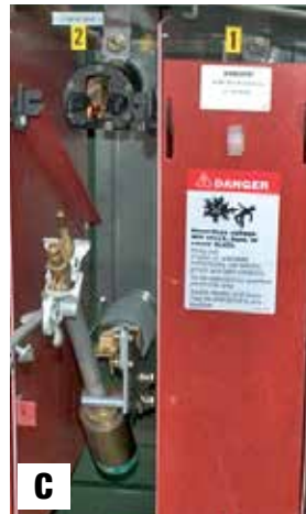
Figure 27. Before opening fuse (a), verify that fuse is latched (b). Place long prong of grappler in pull ring with prongs pointing down. Open/close fuse in a swift non-hesitating motion. And, (d) Reposition grappler with cone in pull ring and prongs cradling fuse. Then, lift fuse up and out of mounting to remove fuse (or lower onto cross bar of hinge if installing fuse assembly).
