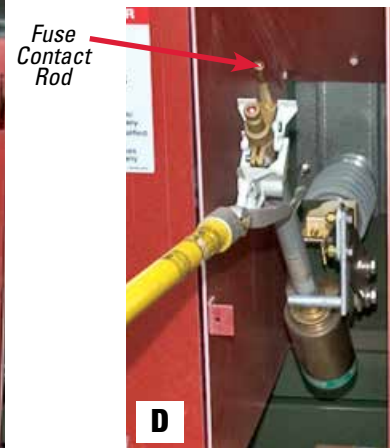
Figure 27. Before opening fuse (a), verify that fuse is latched (b). Place long prong of grappler in pull ring with prongs pointing down. Open/close fuse in a swift non-hesitating motion. And, (d) Reposition grappler with cone in pull ring and prongs cradling fuse. Then, lift fuse up and out of mounting to remove fuse (or lower onto cross bar of hinge if installing fuse assembly).
