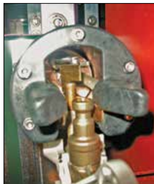
Figure 16. Adjust fuse-hinge assembly when contact rod does NOT engage latch face or latch gap exceeds 1/8".
