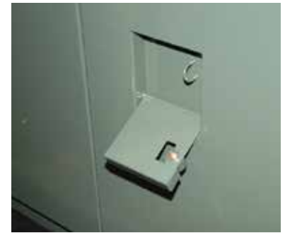
Figure 11. With penta-head bolt fully loosened, handle can be pivoted down to unlatch the door.
