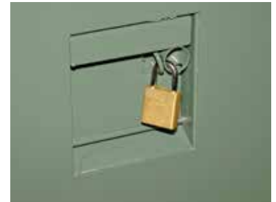
Figure 14. Always close, latch and padlock the enclosure door before leaving the unit or when working on the opposite side.
