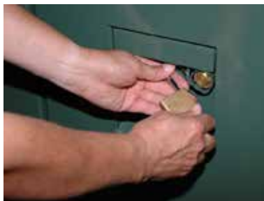
Figure 13. Padlock cannot be inserted until penta-head bolt is fully tightened.
