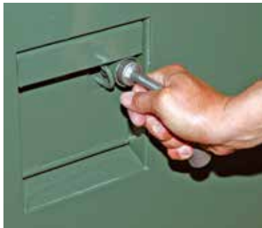
Figure 10. Door handle cover is secured closed by a penta-head (or hex-head) bolt. Turn socket counter-clockwise to loosen bolt.
