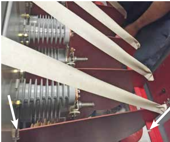
Figure 4. Note how the tab, corner and edge of each switch barrier nests in the appropriate slots in the switch frame and fiberglass barrier support angle.
