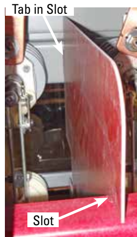
Figure 6. Insert the two tabs on the switch barrier into corresponding slots in the switch frame and insert the slot in the switch barrier into the slot on the fiberglass barrier support angle.
