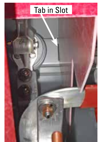
Figure 6. Insert the two tabs on the switch barrier into corresponding slots in the switch frame and insert the slot in the switch barrier into the slot on the fiberglass barrier support angle.
