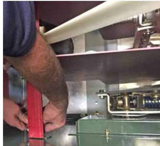
Figure 5. Loosen the hardware that secures the fiberglass angle to the barrier support bracket at each end.
