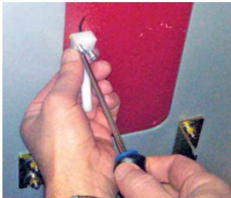
Figure 5. Secure the Ball Socket (with the Ball Rod correctly positioned in it) to the Shutter Barrier by tightening the two screws into the plastic anchors.
