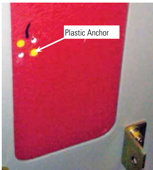
Figure 3. Tap a plastic anchor in the upper-left and lower-right holes of the four holes in the shutter barrier.
