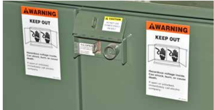
Figure 4. Raise cover to access security bolt. Review and understand the “CAUTION” label on the underside of the cover. Do not use power tools to operate the security bolt.
