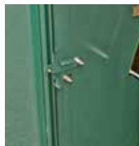
Figure 3. Release passive door by simultaneously pushing on it and raising the latch bracket.
