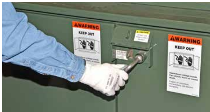
Figure 5. Use a manual wrench with pentahead or hexhead socket as applicable. As explained on the caution label, DO NOT USE POWER TOOLS . Rotate the security bolt clockwise or counter-clockwise to release three-point latch and charge for subsequent door closing.
