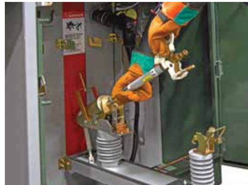
Figure 6. Alternate method using insulating-gloved hand, if user's standard operating procedures permit, to remove or install fuse assembly of fuse mounting.
