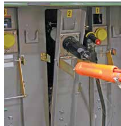
Figure 2. Fuse mounting being lowered to access fuse (or raised to reinstall fuse).
