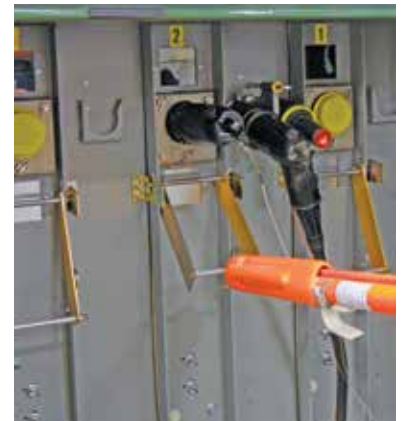
Figure 1. Interlock lever being raised to unlocked position (or lowered to locked position).
