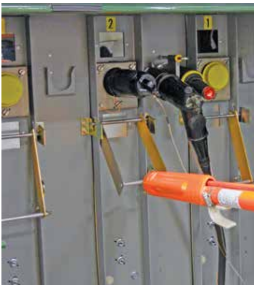
Figure 24. Interlock lever being raised to unlocked position (or lowered to locked position).
