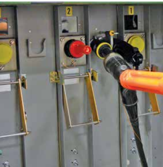
Figure 21. Shotgun clamp stick secured to elbow with elbow moved to feed through standoff bushing on parking stand.
