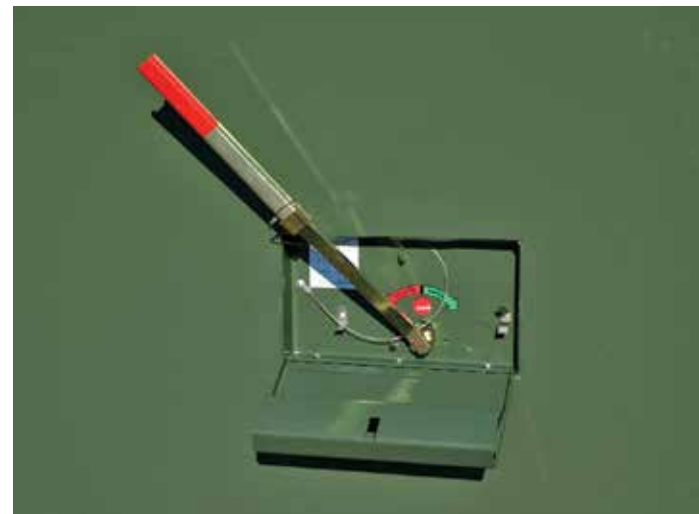
Figure 15. Place operating handle on hex shaft of switch. Rotate handle in desired direction as shown by switch position indicator.
