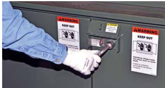
Figure 6. Use a manual wrench with pentahead or hexhead socket as applicable. As explained on the caution label, DO NOT USE POWER TOOLS . Rotate the security bolt clockwise or counter-clockwise to release three-point latch and charge for subsequent door closing. Do not use power tools to operate the security bolt.
