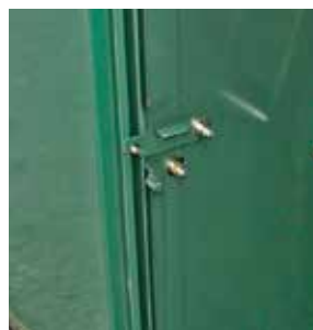
Figure 4b. Release passive door by simultaneously pushing on it and raising the latch bracket.
