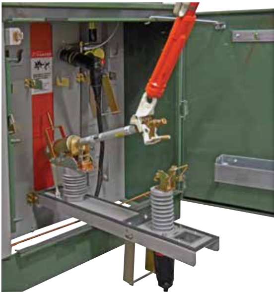
Figure 28. By pulling shotgun clamp stick upward, fuse will unlatch.
