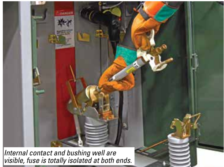
Figure 30. Alternate method using insulating-gloved hand, if user's standard operating procedures permit, to remove or install fuse assembly of fuse mounting.
