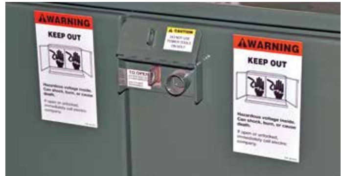
Figure 5. Raise cover to access security bolt. Review and understand the "CAUTION" label on the underside of the cover.
