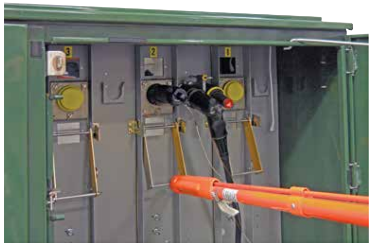
Figure 23. Shotgun-clamp stick secured to interlock lever.
