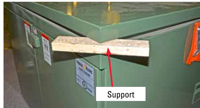
Figure 4a. Wood block support installed at corner, initial location.
