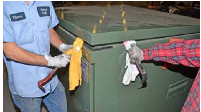
Figure 3. Using pry bars to "break loose" the roof gasket attachment. Protective measures, such as wrapping the pry-bars with cloth as shown should be used to protect enclosure finish (paint).
