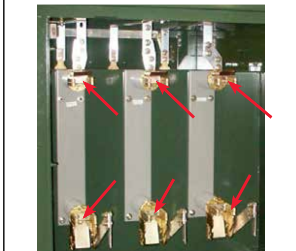
Figure 2. Lubrication points on load-break fuse mounting (at top) include three contact locations, namely, the main contact, forward contact and fuse hinge contacts. Two lubrication points on non-load-break fuse mountings (above).
