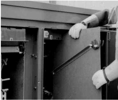
Figure 8. Switch and fuse side removable barriers facilitate cable installation and termination when the switchgear is de-energized. Fuse side is shown. Lift up until rivets on barrier align with slot in top front barrier guide, and pull out to remove barriers.
