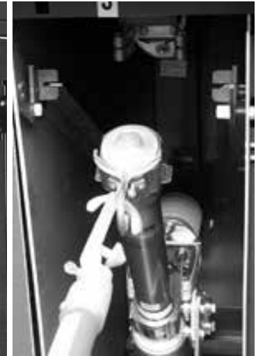
Figure 20. With the fuses de-energized, open/close fuses using a grapppler tool. Fuses should be removed using a large clamp, following fuse manufacturer's instructions.
