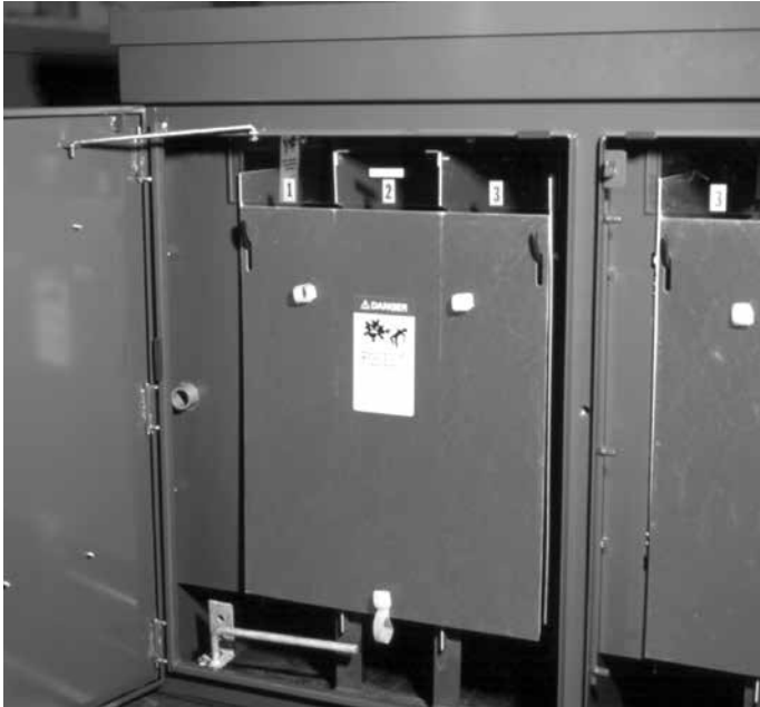
Figure 17. Switch DP barrier shown in normal hanging position.
