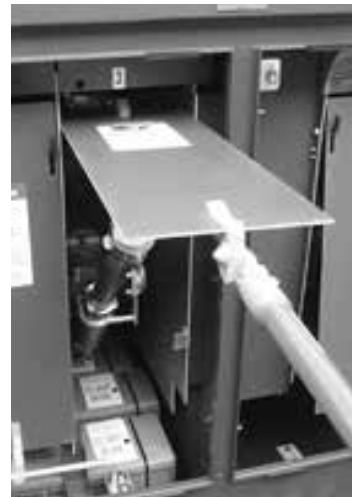
Figure 21. Install fuse DP barrier.
