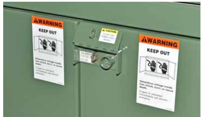
Figure 3. After removing padlock, raise cover to access security bolt.
