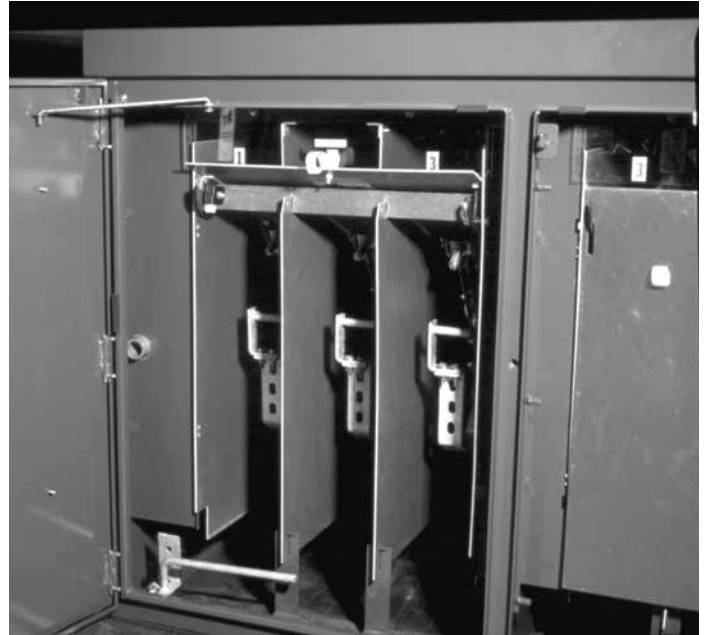
Figure 18. Switch DP barrier in slide-in position.
