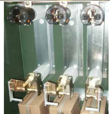
Figure 2. Lubrication points on fuse mounting include three contact locations, namely, the main contact, forward contact and fuse hinge contacts.
