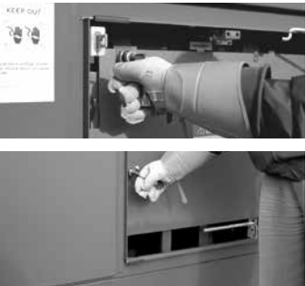
Figure 9. Disengage barrier security bolt.
