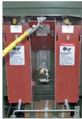
Figure 21b. Use long prong on grapple tool to remove fuse DP barrier from slide-in position.
