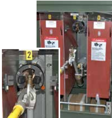
Figure 20. Open/close fuse in a swift non-hesitating motion.
