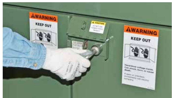
Figure 4. Use standard pentahead socket (or hexhead socket if optional hexhead bolt is specified) to turn bolt. Rotate security bolt clockwise or counter-clockwise to release three-point latch and charge for subsequent door closing. Do not use power tools to operate the security bolt.
