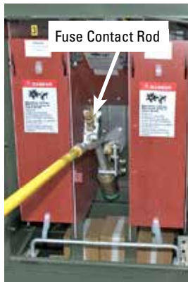
Figure 22. Reposition grapple with cone in pull ring and prongs cradling fuse. Then, lift fuse up and out of mounting to remove fuse (or lower onto cross bar of hinge if installing fuse assembly).
