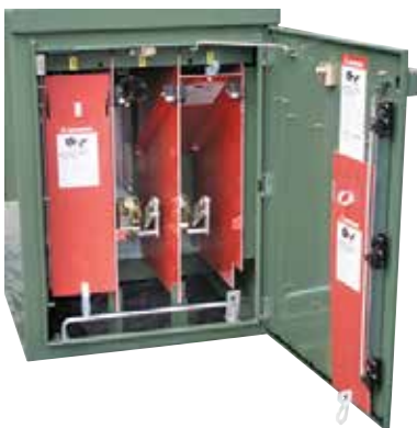
Figure 21c. Barrier may be temporarily stored on door with edge behind latch operating link and bottom resting in flange of door.
