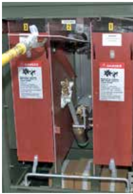
Figure 21a. Position lower hoop of DP barrier onto cone of grapple with barrier supported by prongs on grapple.
