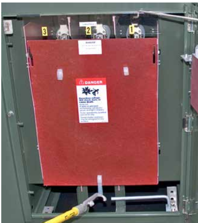
Figure 17. Switch DP barrier shown in normal hanging position. With switch open, grip bottom ring on barrier with grappler tool to raise and lower into slide-in position.
