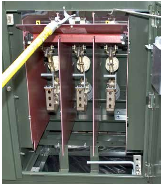
Figure 18b. Lower switch DP barrier to slide-in position. Remove barrier using grappler inserted in barrier hoop - pull up, drawout and lower onto hooks.
